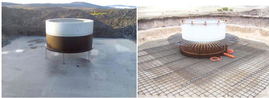
Plate 2-1: Levelled turbine tower “can” Plate 2-2: Steel reinforcement being added
